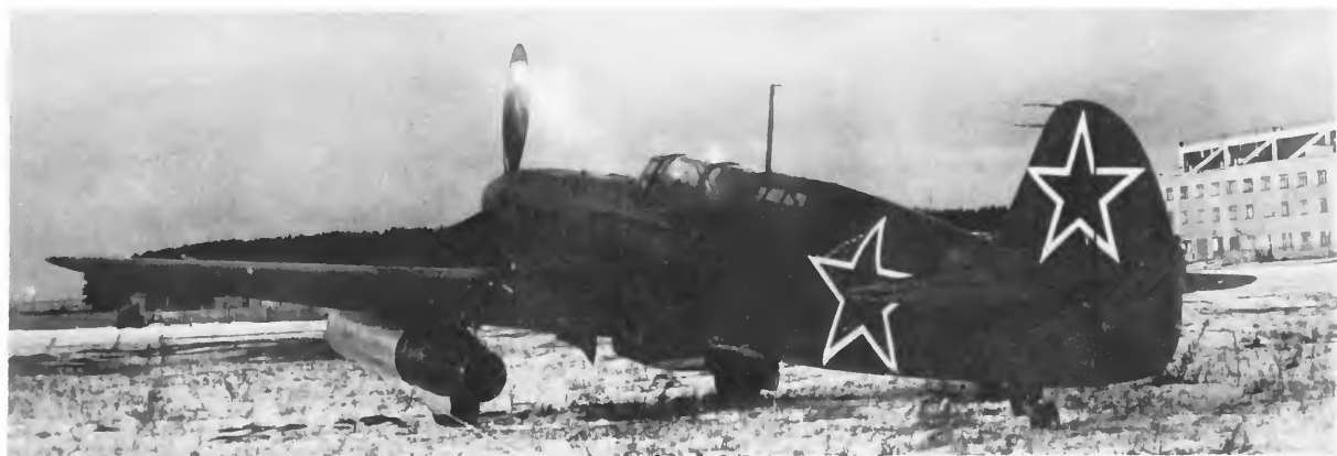
FIGURE 4.—DM-4 ramjet engines mounted beneath wings of A. S. Yanovlev aircraft Yak-7b to supplement performance.
