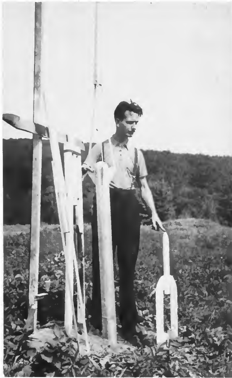
FIGURE 13.—H. F. Pierce, with solid-fuel rockets of various designs tested by the Committee to determine the best aerodynamic shape and other characteristics of high-altitude rockets. These tests took place principally at a site near Pawling, New York, where this picture was taken in 1935, during one of the earliest series. These rockets and those in Figure 14, were constructed by various members of the Experimental Committee and were powered by commercial 4-pound and 6-pound skyrocket motors.
