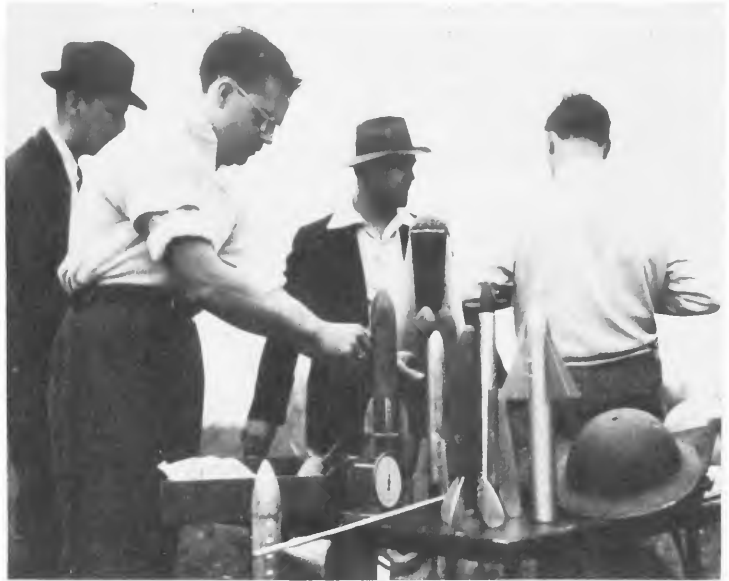
FIGURE 13.—H. F. Pierce, with solid-fuel rockets of various designs tested by the Committee to determine the best aerodynamic shape and other characteristics of high-altitude rockets. These tests took place principally at a site near Pawling, New York, where this picture was taken in 1935, during one of the earliest series. These rockets and those in Figure 14, were constructed by various members of the Experimental Committee and were powered by commercial 4-pound and 6-pound skyrocket motors.
